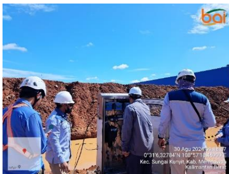
Gambar 2. Proses Instalasi PH Analyzer
